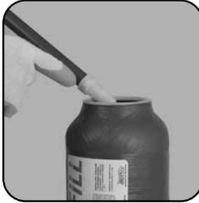
Pull the connection fitting with the riser tube upwards.
